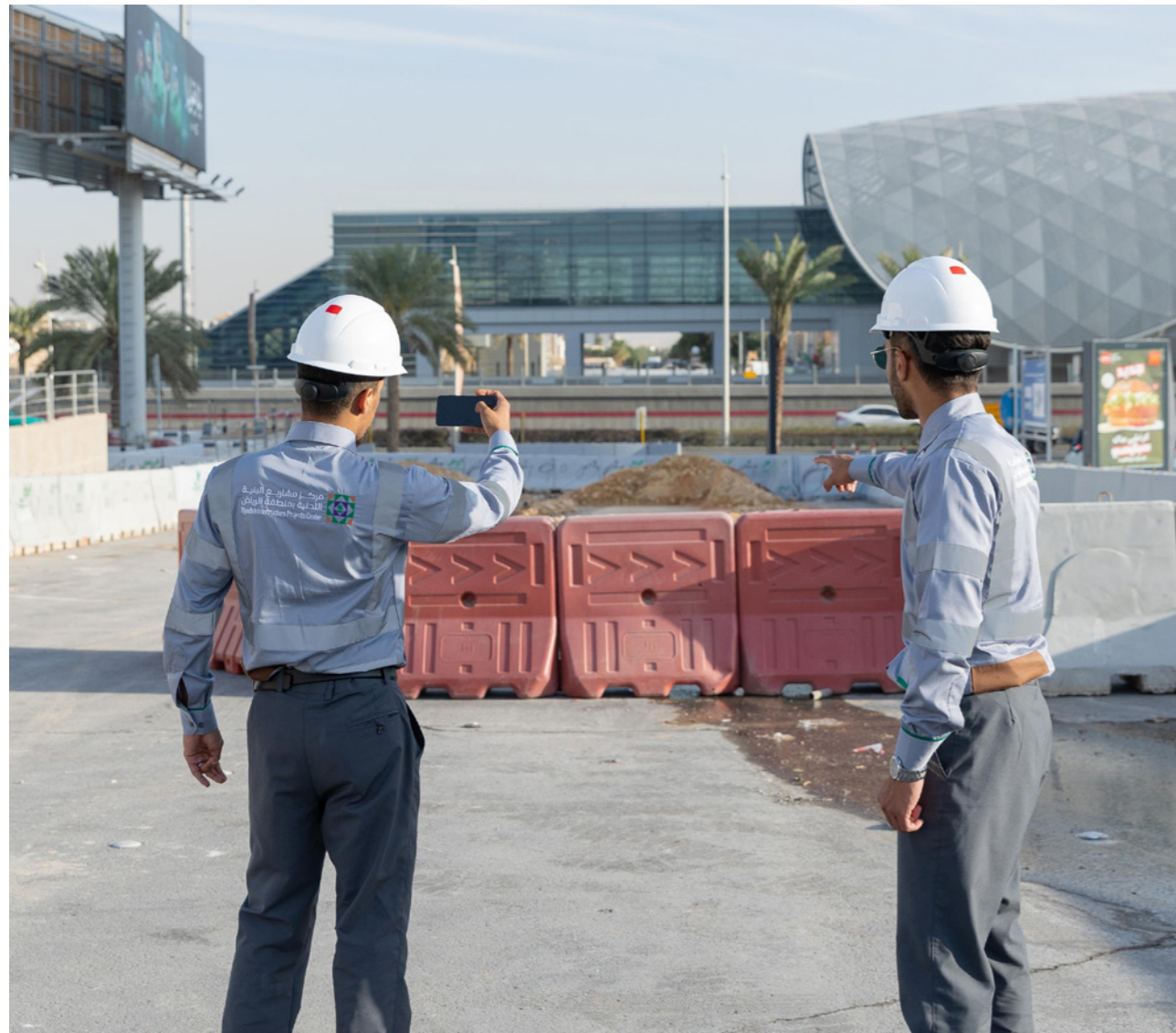
Infrastructure Projects Code, Riyadh, Saudi Arabia ©2025 RIPC
