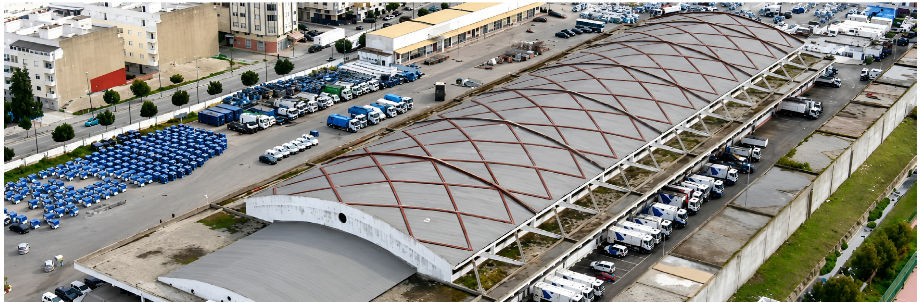
project for repurposing and rehabilitating the old wholesale fruit and vegetable market in Tangier and transforming it into a regional space for exhibitions and arts ©2026 City of Tangier
