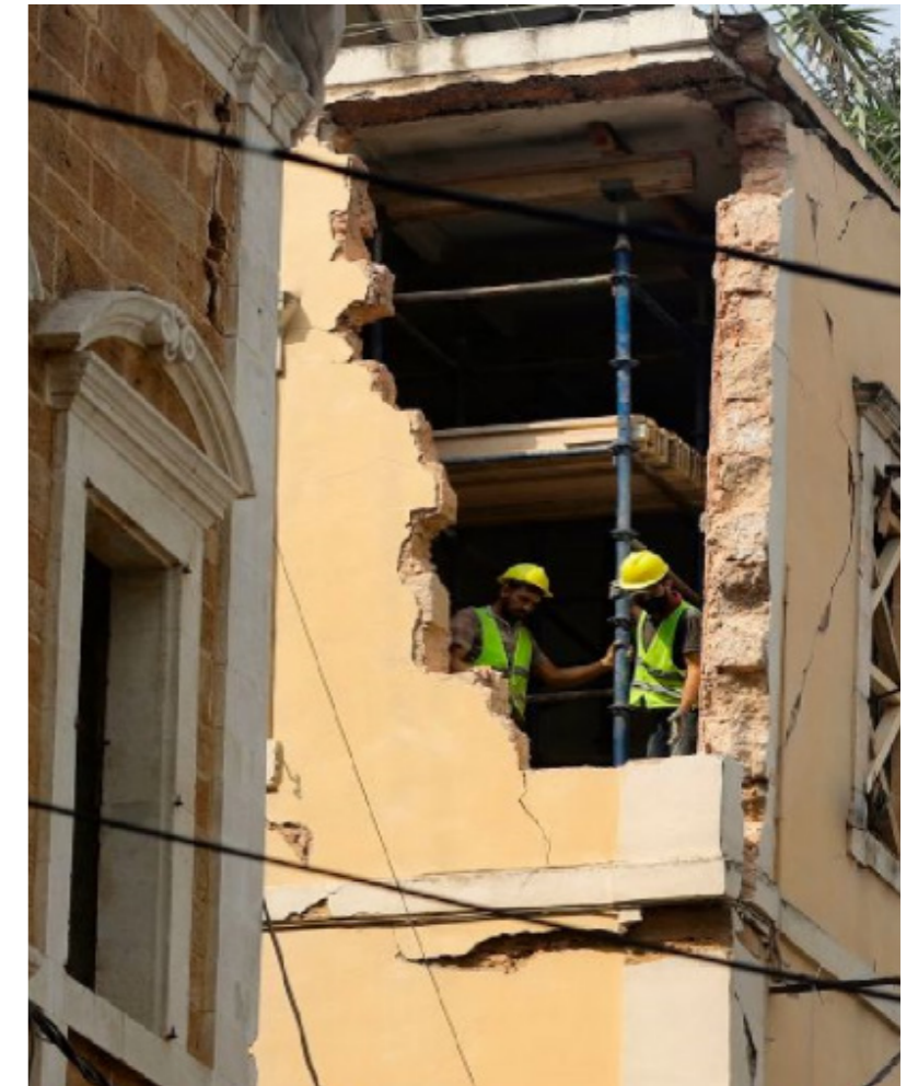
Workers restoring a blast-damaged heritage building, Beirut, Lebanon ©2021 The New Arab
