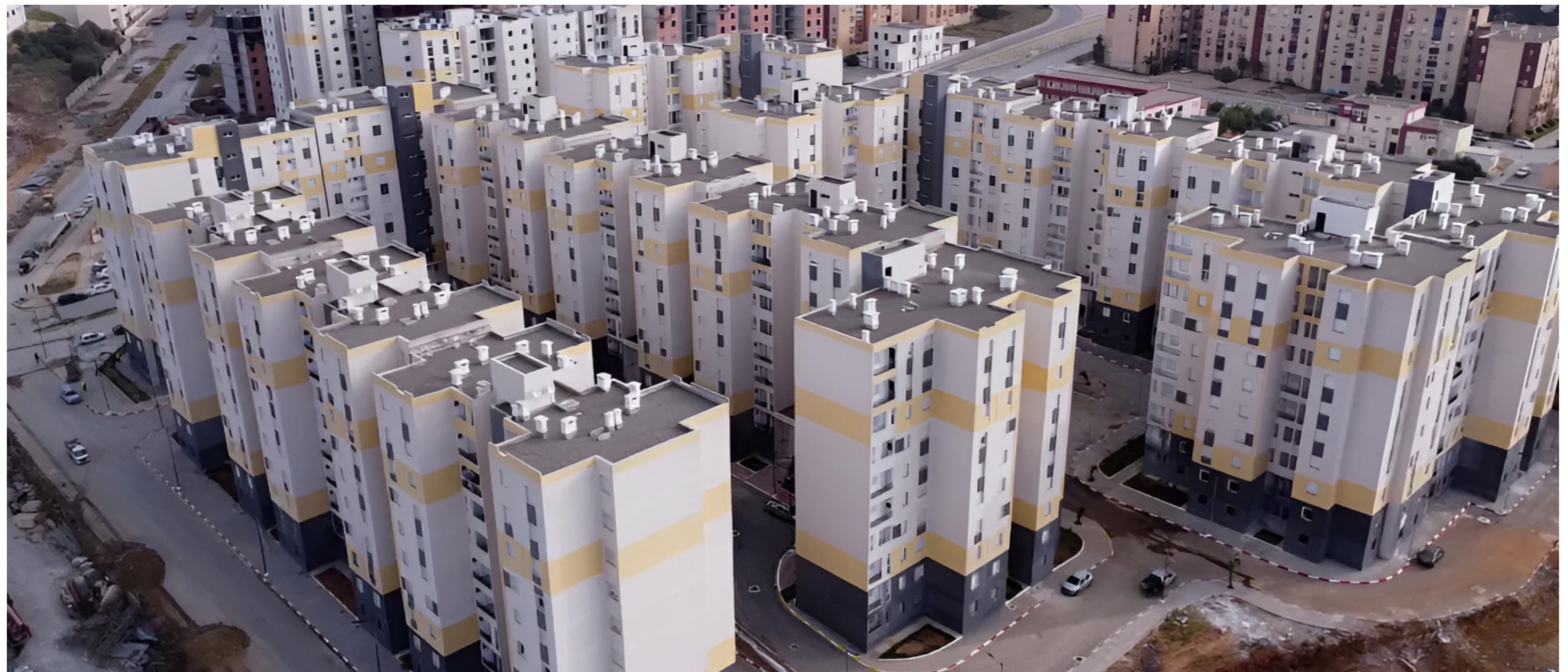
AADL 2 housing units ©2025 UltraAlgeria
