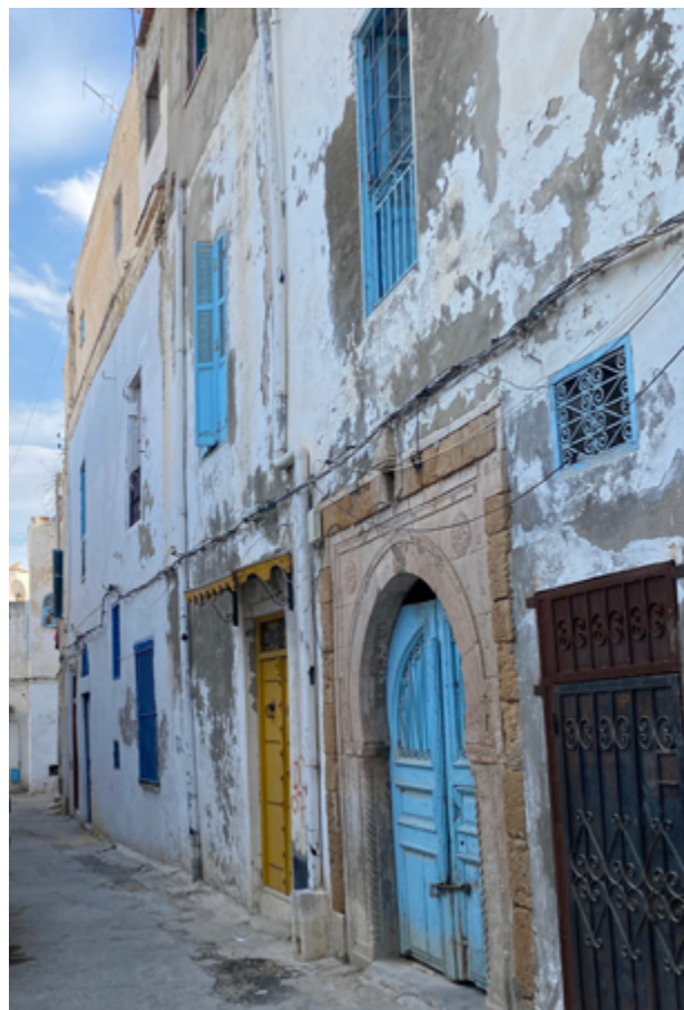
Figure 3.16: Visible decay on an ancient residential building's facade in the Medina © Authors, 2024
