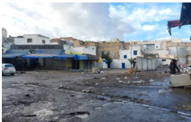
Figure 4.3: Rainwater accumulated on impermeable ground © Authors, 2024
