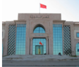
Municipality includes lighting, vegetation, and waste units
