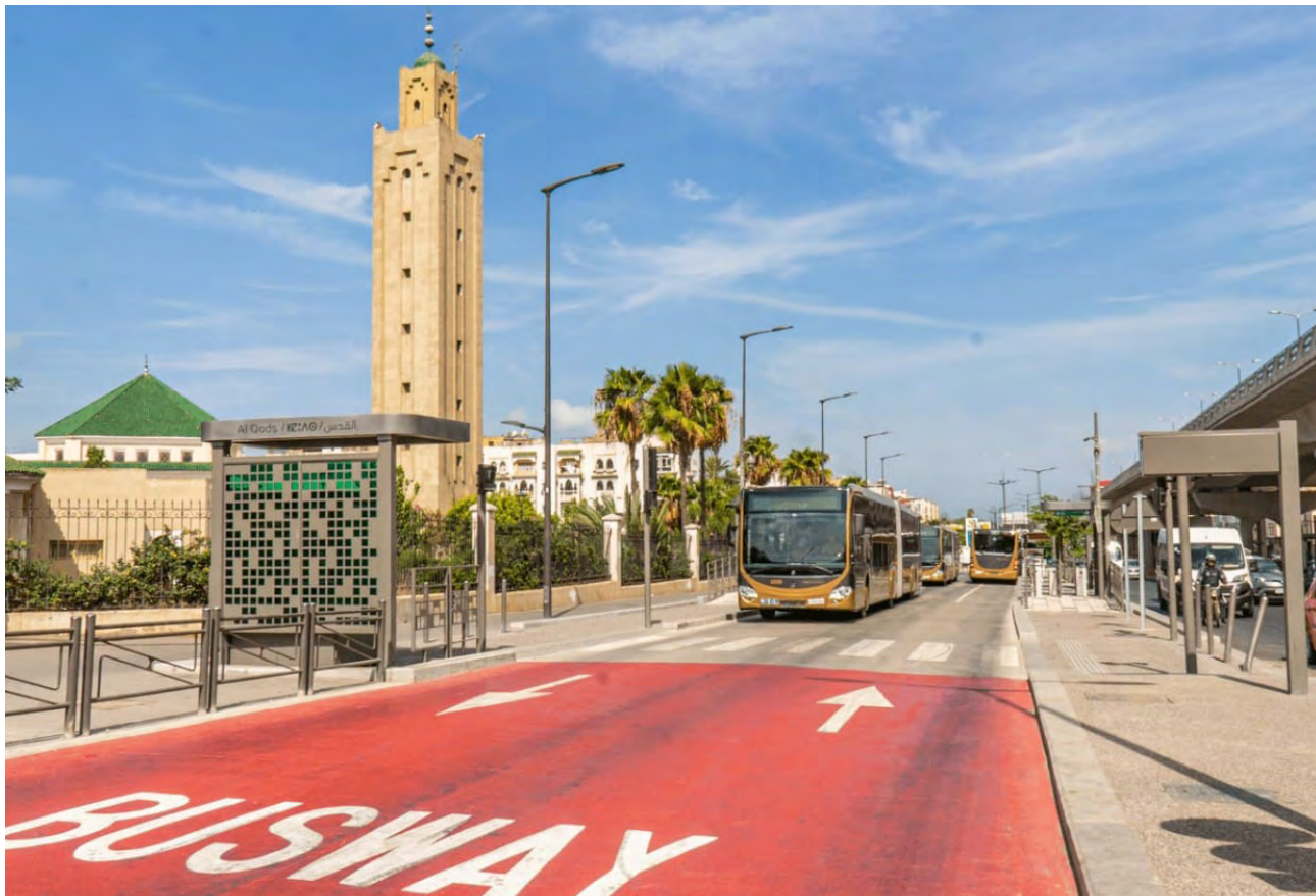
Busway ©2024 Municipality of Casablanca
