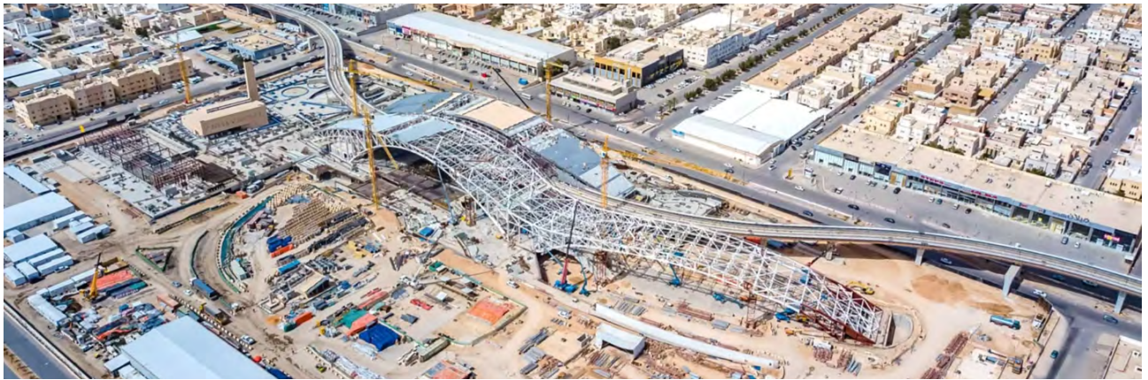
Riyadh Metro: Western Station ©2024 RCRC
