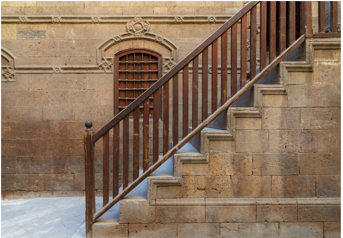
Photo: Staircase with wooden balustrade leading to Zeinab Khatoun historic house, Darb Al-Ahmar ©2024 Halit Sadik | Shutterstock
