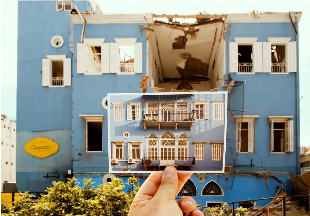
Photo: Buildings affected by the Beirut port explosion ©2024 Joseph M Khoury | @joekhourystudio | Project@bouyoubeirut
