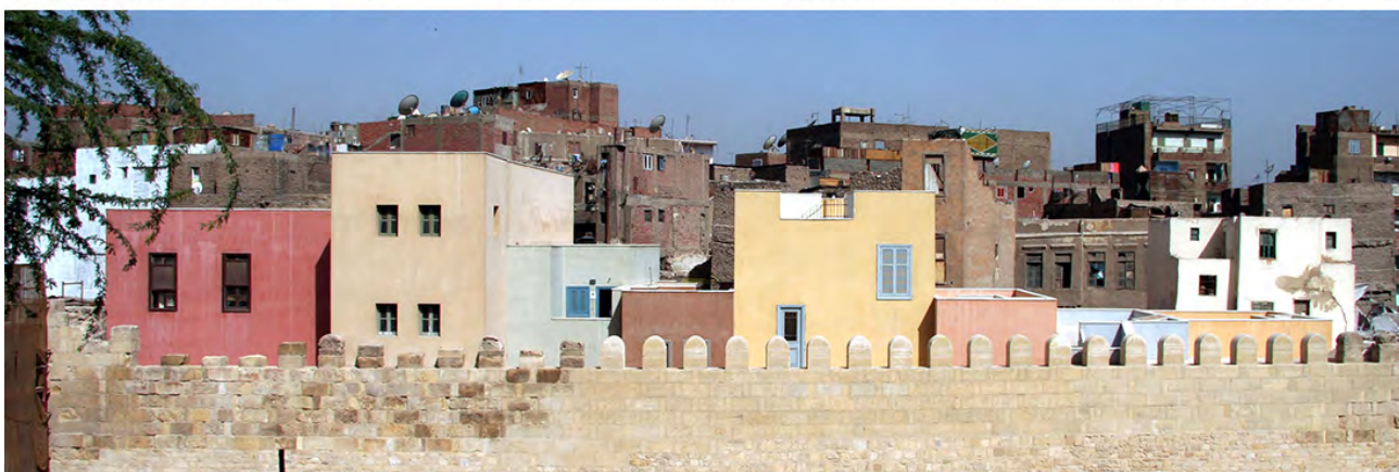
Photo: Before (above) and after (below) the Darb al-Ahmar Housing Rehabilitation Program © 2024 Tadamun
