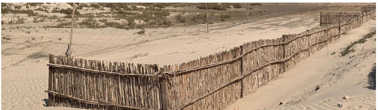
Photo: Reed Fencing - Kafr El Sheikh UN-Habitat, ©2022
