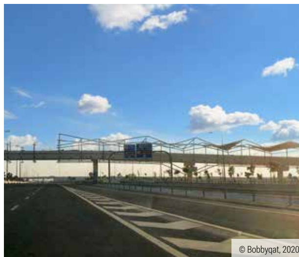
Figure 4.66: Al Khor Coastal Road in Al Heedan, Qatar.
