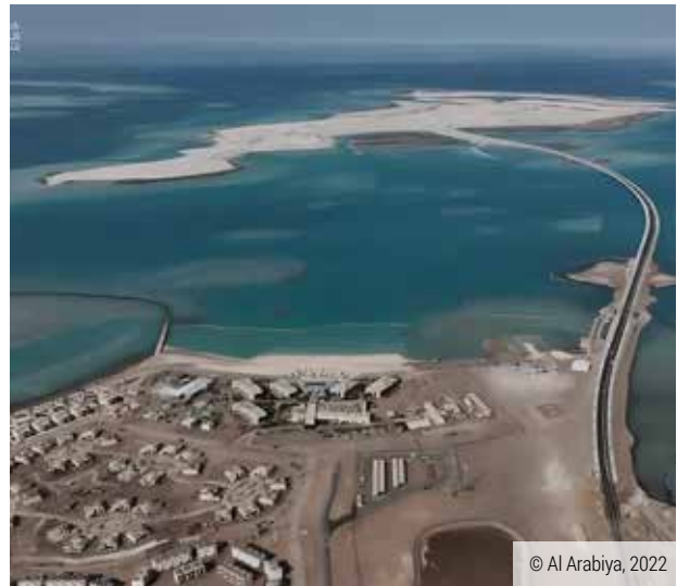
Figure 4.118: Construction works on the Shura and Shura Bridge project in Saudi Arabia.
