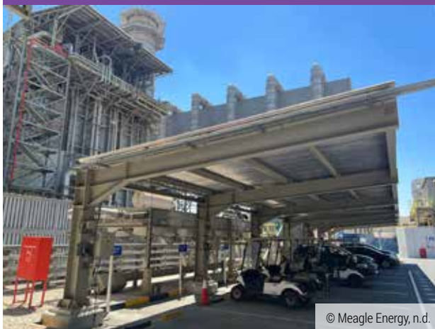
Figure 4.81: Solar-powered EV charging station at ALBA Factory, Bahrain.
