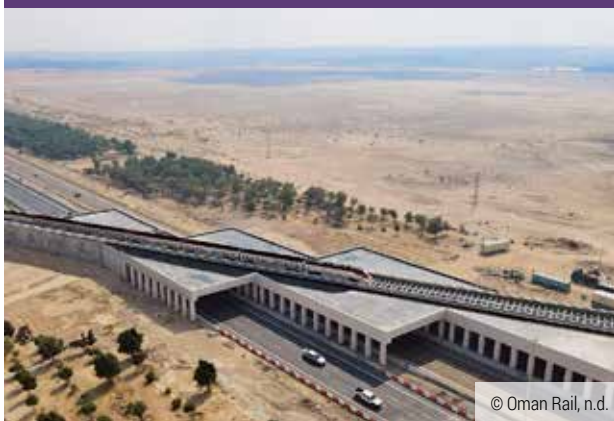
Figure 4.61: Part of The UAE and Oman 303-kilometer rail network.
