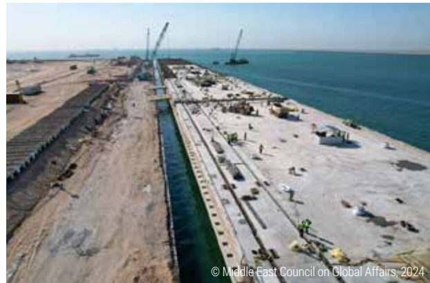
Figure 4.38: Construction of Iraq's Development Road Project.
