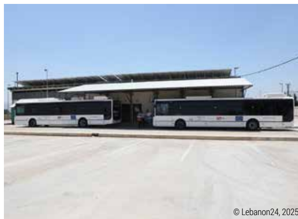
Figure 4.50: dedicated station in Zahle that is the hub for the city's new bus network for organized urban mobility.
